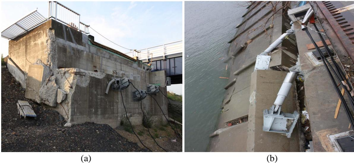
Figure 2 Fall-off prevention devices tore off by tsunami waves;
