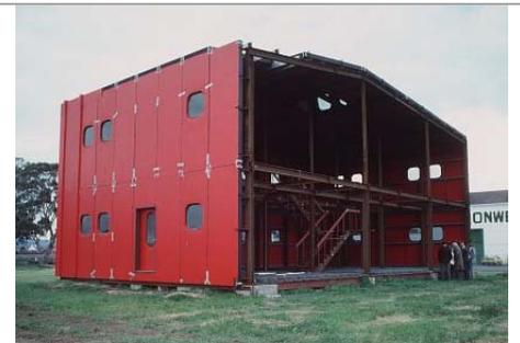
**Figure 10 (above):** Trial erection of the Mawson living Quarters in Melbourne in 1988
