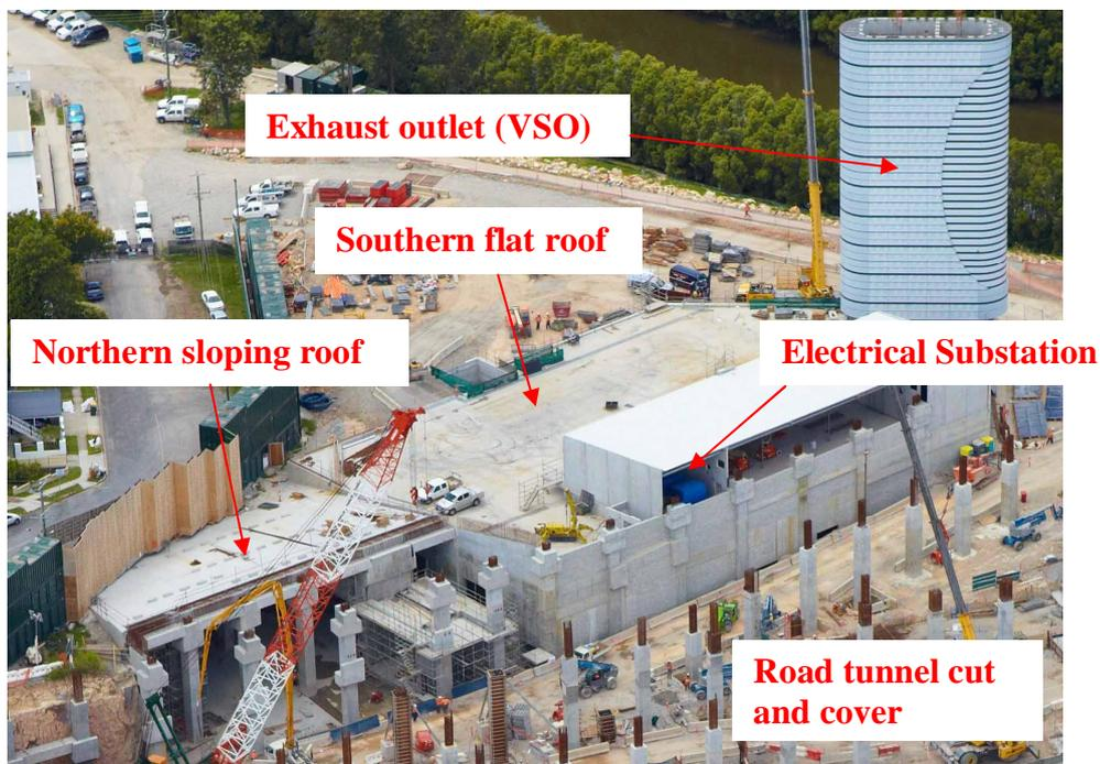
**Figure 3.** An aerial view of Bowen Hills Ventilation Station in Construction
